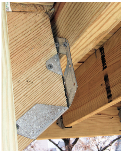
Figure 4. Every hole of a piece of framing hardware must be filled with the proper nail or structural screw.
