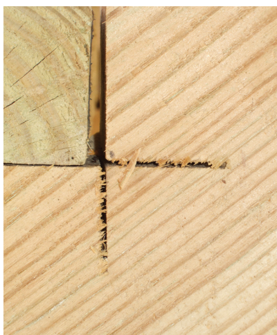
Figure 7. Overcuts weaken stringers and reduce the uncut portion to less than the code-required 5 inches.
